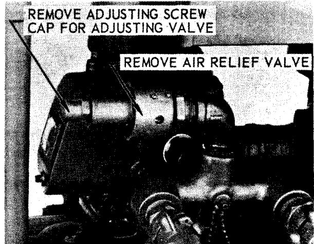
A. AIR-RELIEF VALVE REMOVAL
